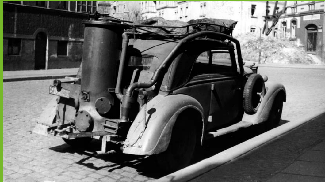
Engine powered by wood combustion instead of fuel
